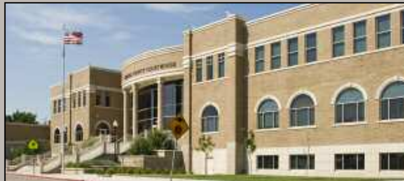
The Chaves County Courthouse.
