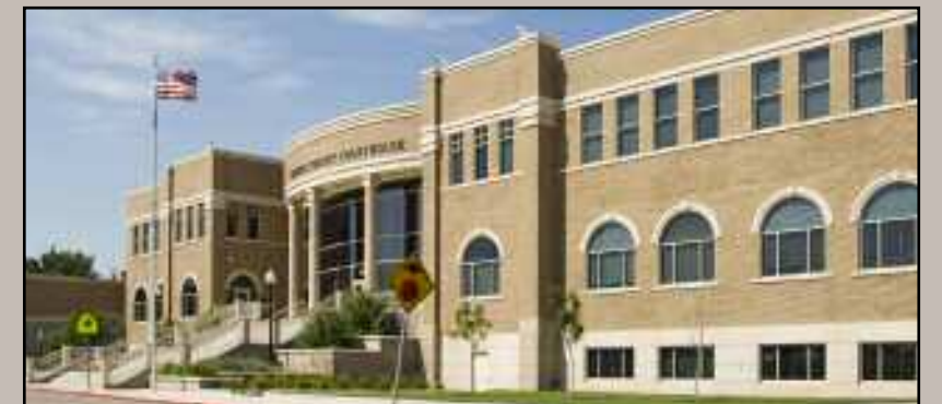
The Chaves County Courthouse.
