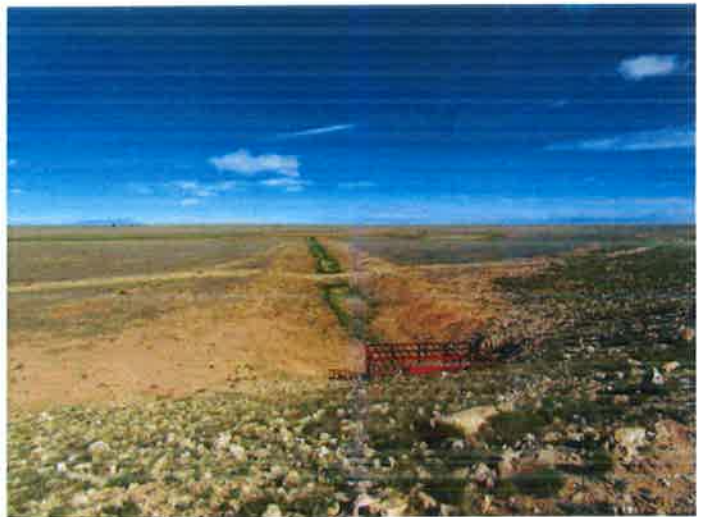
RIGHT: View of a control gate used to control water flow out of the dirt banks during periods of heavy rainfall.
